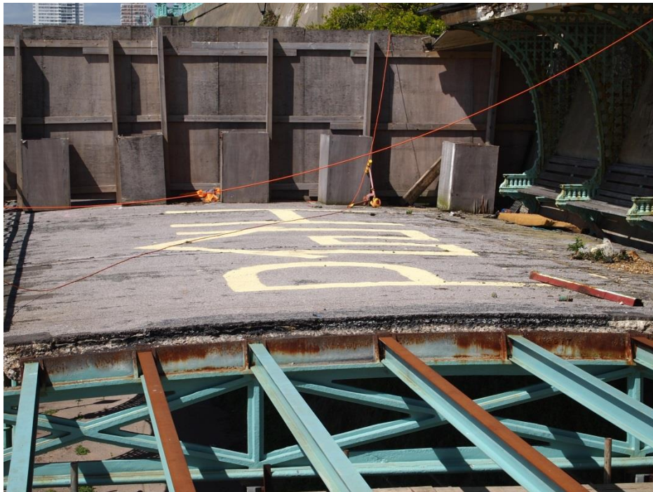
Figure 4.1 – Steel I-beams with concrete jack arches removed
