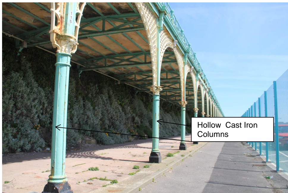
Figure 4.12 – Cast iron columns
