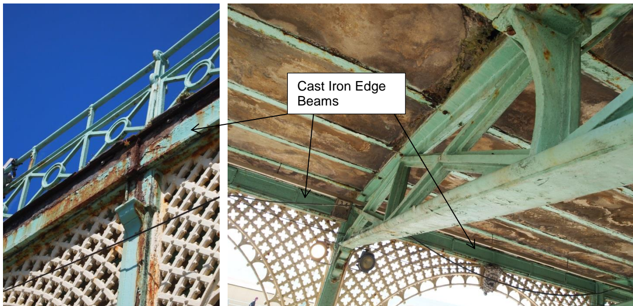
Figure 4.7 – Cast iron edge beam
