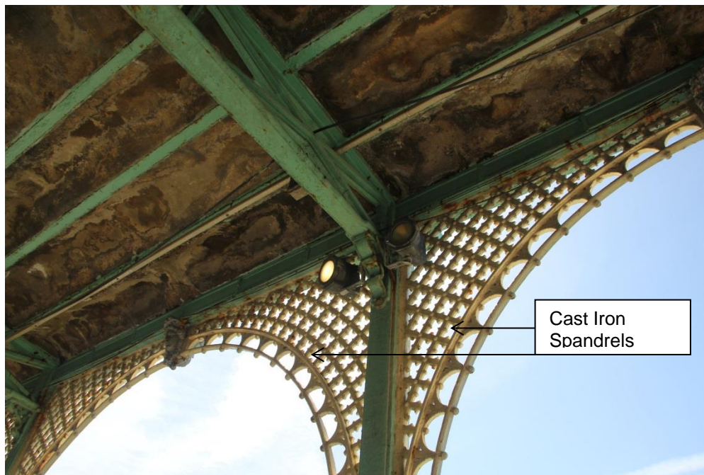
Figure 4.11 – Cast iron spandrels
