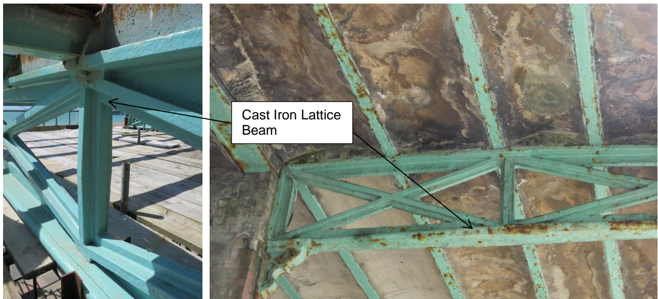
Figure 4.5 – Cast iron lattice beams
